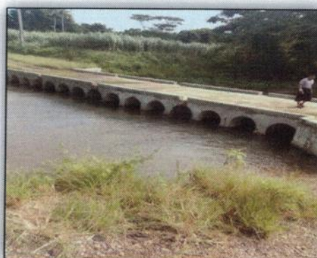
Figures 3& 4: Uluisila Crossing before and after construction of Irish Crossing
